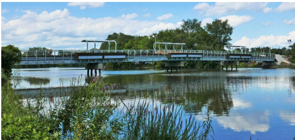
Footbridge over the Hackensack River
